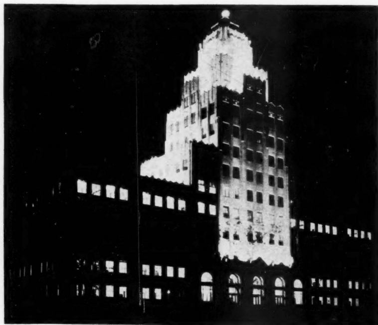
This factory building of the Staley Company, Decatur, Ill., has its elaborate color-changing floodlighting controlled by three-element mercury tubes. Two hundred projectors are employed
